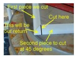
The black mark in this photo is where the cut will be made. The small triangular shape to the left is our return. When cutting this on the miter saw be careful as the small piece may fly off.
