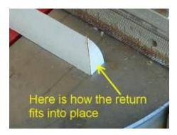
The return fits together with the extremity of the quarter round that will be installed. The return needs to be glued on with a good adhesive caulk or some wood glue. After the piece is installed use some caulk to fill in any gaps that may show.
